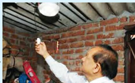
*Photo-Voltaic Integrated Micro Solar Dome (MSD)*
